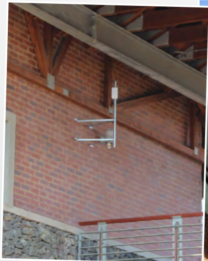
Wireless Antenna Installation
