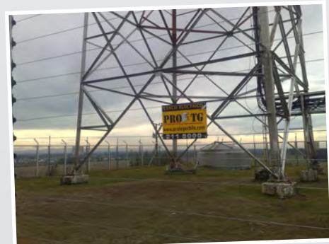
Power Station, Chili
