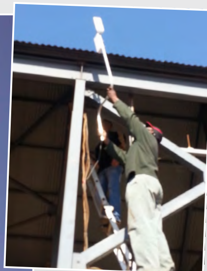
Wireless Repeater at Entrance
