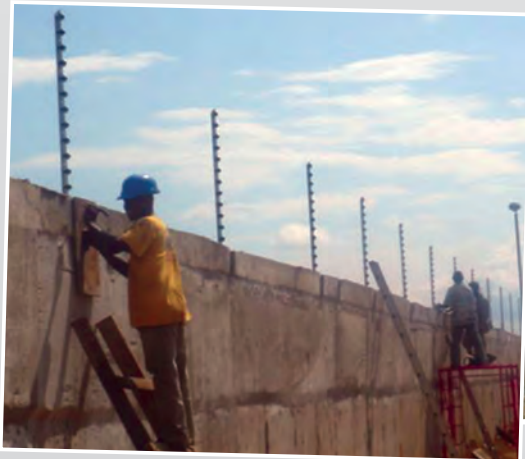
Security fence installation, India
